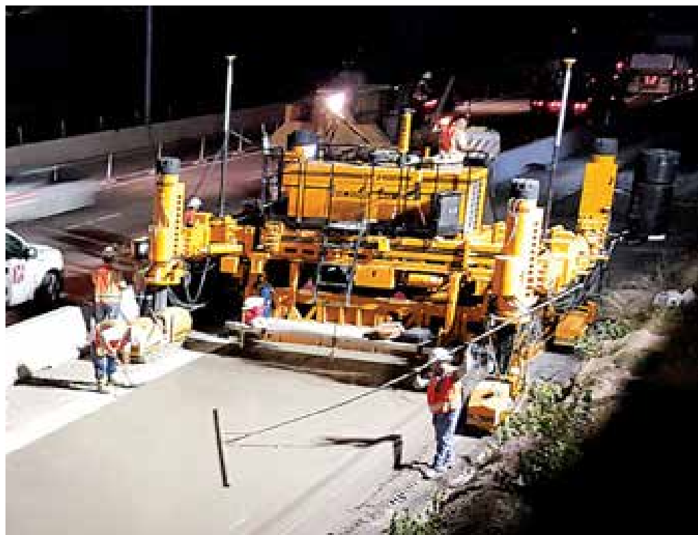
The GOMACO four-track GP-2400 scabs on a single lane with an integral curb on the right side during a night pour using 3D machine guidance.
