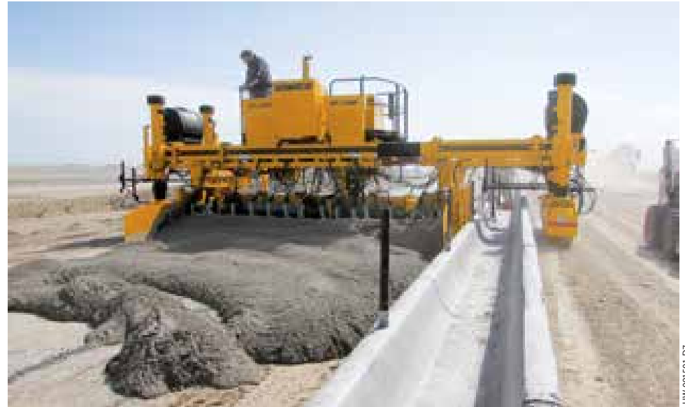
A two-track GP-2400 is slipforming a dairy pad against the existing feed bunk. The left end frame and leg straddle the feed bunk, and sonic sensors are being used within the bunk for grade.
