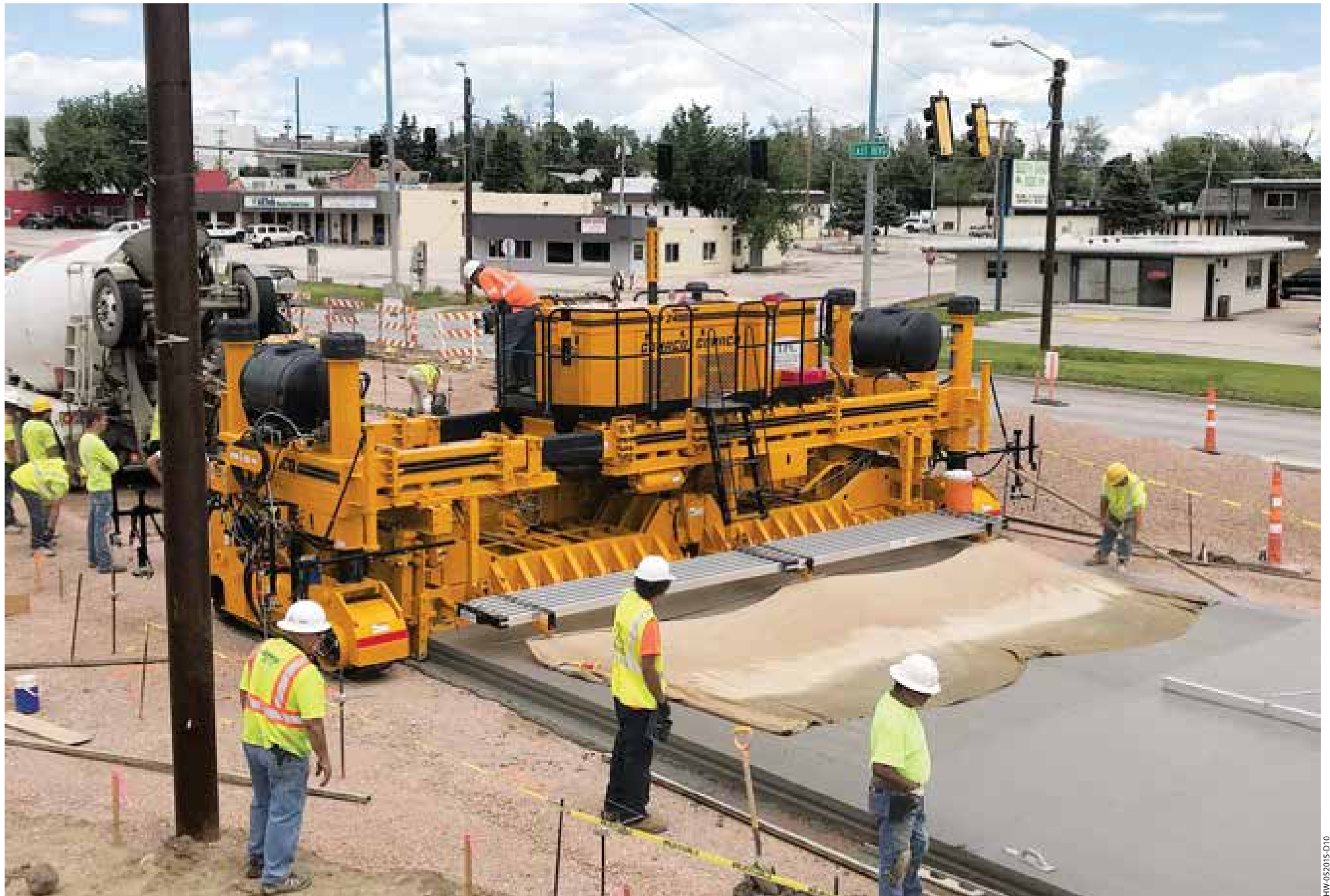
The GP-2400's ability to pave up to 24 feet (7.3 m) wide in tight, urban conditions makes it an ideal municipal paver. A two-track GP-2400 slipforms this new city street with a female keyway, in between existing obstacles.
