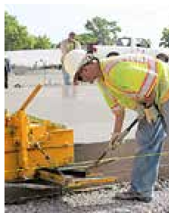
When the slipforming begins, the trailing form is lowered and the manual bar insertion resumes.
