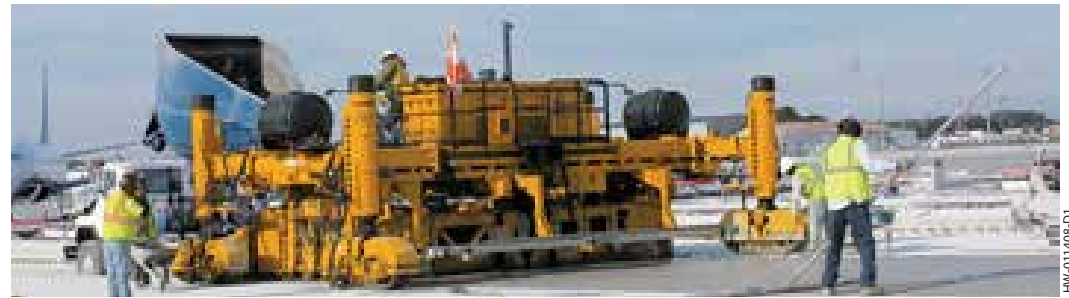
A GP-2400 featuring a 5400 series mold with two telescoping end sections, end slump adjustment, and a self-supported PTA paves a new airport ramp.
