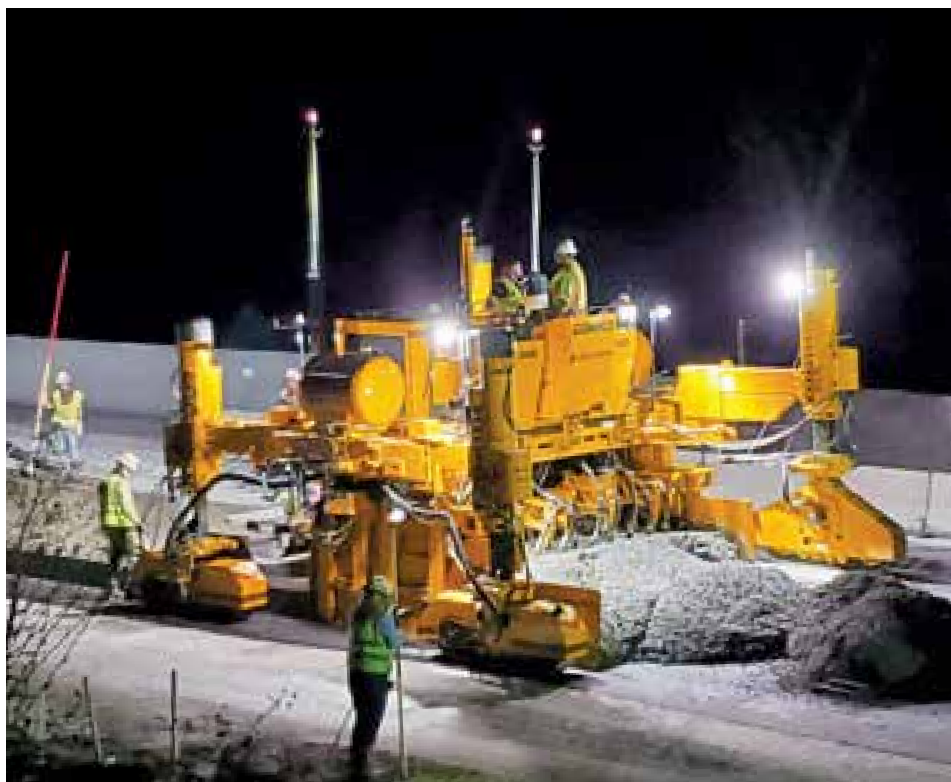
A GOMACO four-track GP-2400 slipforms a highway using 3D machine guidance. The left side is using high-rise tracks that are only six inches (152 mm) wide to achieve minimum clearance.
