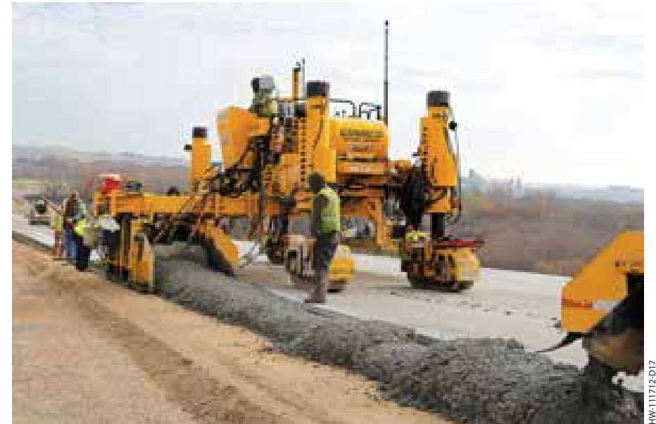
The GP-2400 with a sidemounted mold paves scab-on shoulder using 3D machine guidance.
