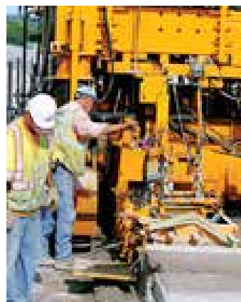
When the slipforming begins, the trailing form is lowered and the manual bar insertion resumes.
