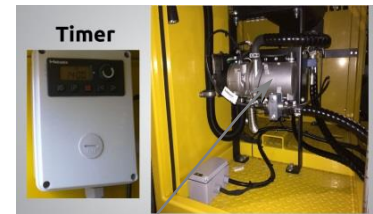
HEATING SYSTEM FOR LUBE OIL TANK
